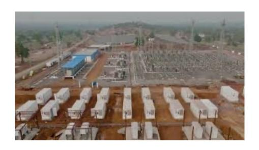
This Delhi BESS is South Asia's largest utility-scale system and India's first commercially approved energy storage system. It has a total storage capacity of 40 Megawatt-hours (MWh). It uses Lithium Iron Phosphate (LFP) technology, which is safe, stable, and works well in Delhi's climate
